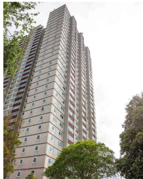
Left: Cool façade materials could be considered for Park Towers Photo: Mark Stewart / News Corp Australia
