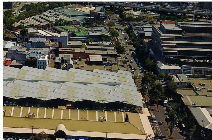
Below: Large exposed roofs of the business, retail and industrial areas of the South Melbourne Study Area Photo: Bob Tan / Wikimedia / CC BY-SA 4.0
